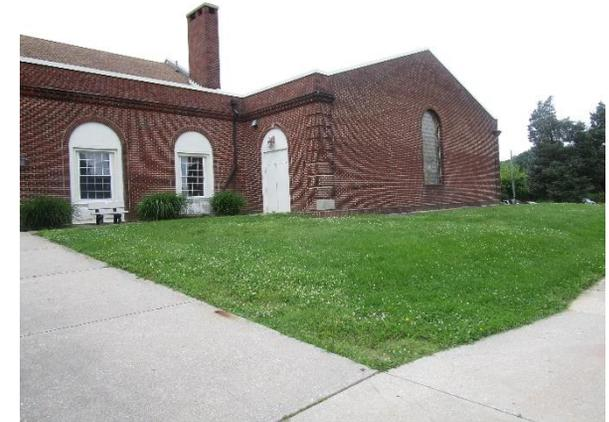
Bioretention systems can be installed in the turfgrass areas in the front of the building. Bioretention systems can capture, treat, and infiltrate rooftop runoff. A preliminary soil assessment suggests that more soil testing would be required before determining the soil's suitability for green infrastructure.
