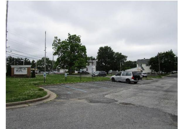
Parking spots at the entrance of the building can be replaced with pervious pavement which will capture and infiltrate stormwater from the parking lot. A bioretention system can be installed at the front of the building to capture runoff from the rooftop. A preliminary soil assessment suggests that more soil testing would be required before determining the soil's suitability for green infrastructure.
